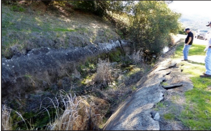
Cracks and separated lining in the canal
