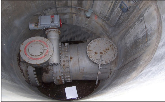
Typical steel pipeline in line valve vault
