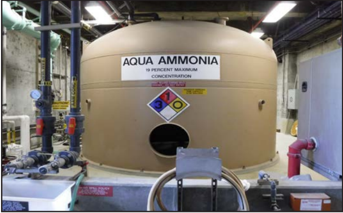
Rinconada Water Treatment Plant Aqua Ammonia Tank
