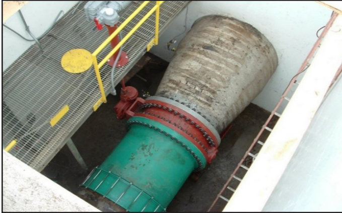
New line valves, actuators, and vaults similar to this will be installed along the East, West, and Snell pipelines
