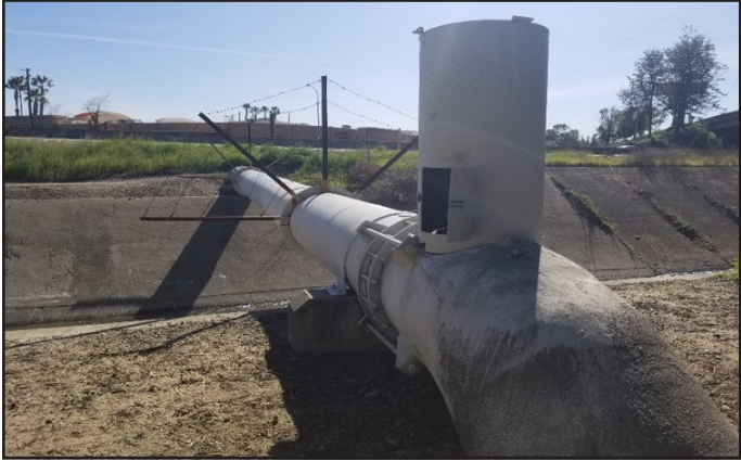
A typical air release valve within the project scope
