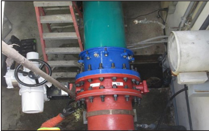
A typical rehabilitated line valve assembly
