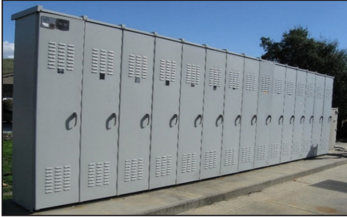
Motor control center switchboard
